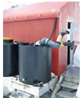
Gary fixing a water tank at a mountain hut
