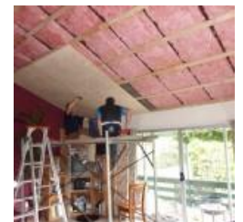
Insulating the base
